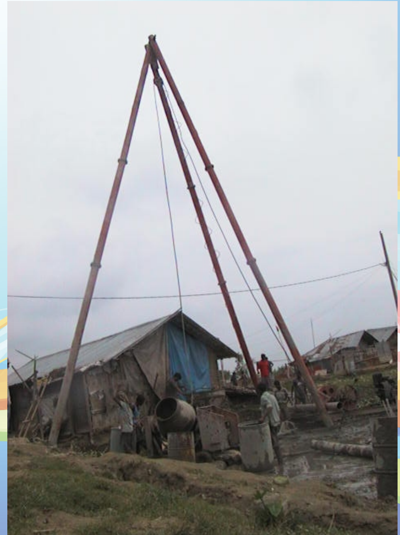
PILLING WORK FOR 132 kV TRANSMISSION LINE AT CHITTAGONG
