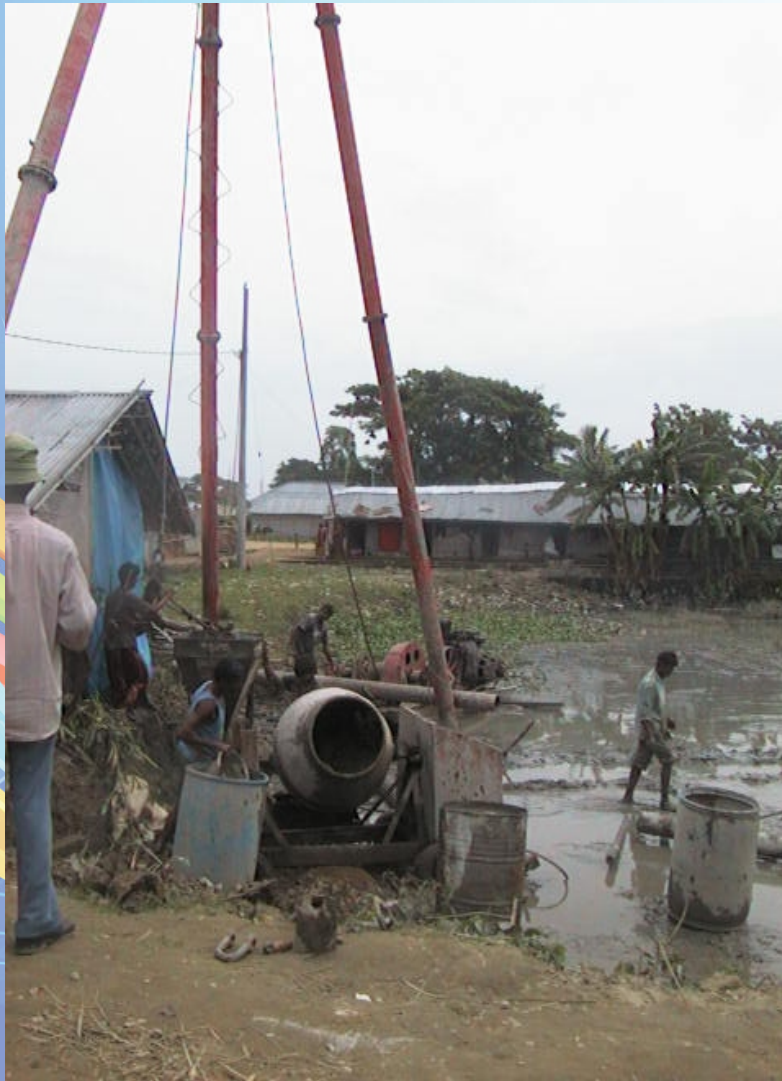
PILLING WORK FOR 132 kV TRANSMISSION LINE AT CHITTAGONG
