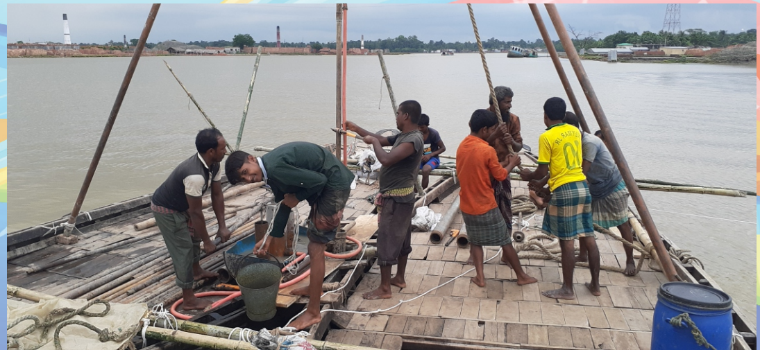
OFFSHORE BORING FOR CIRCULAR ROAD, KHULNA
