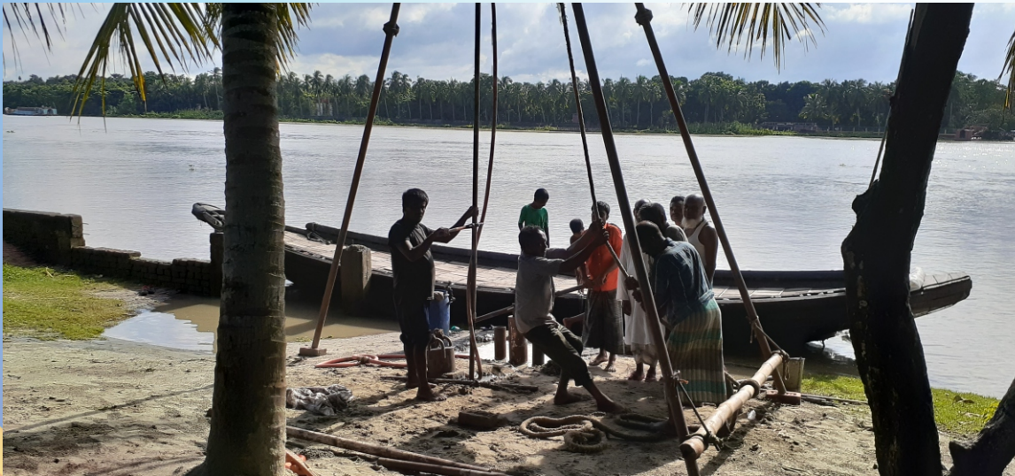
ONSHORE BORING FOR CIRCULAR ROAD, KHULNA
