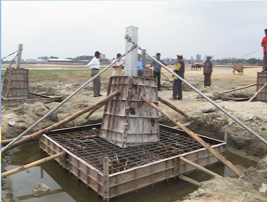
FOUNDATION WORK FOR TRANSMISSION LINE
